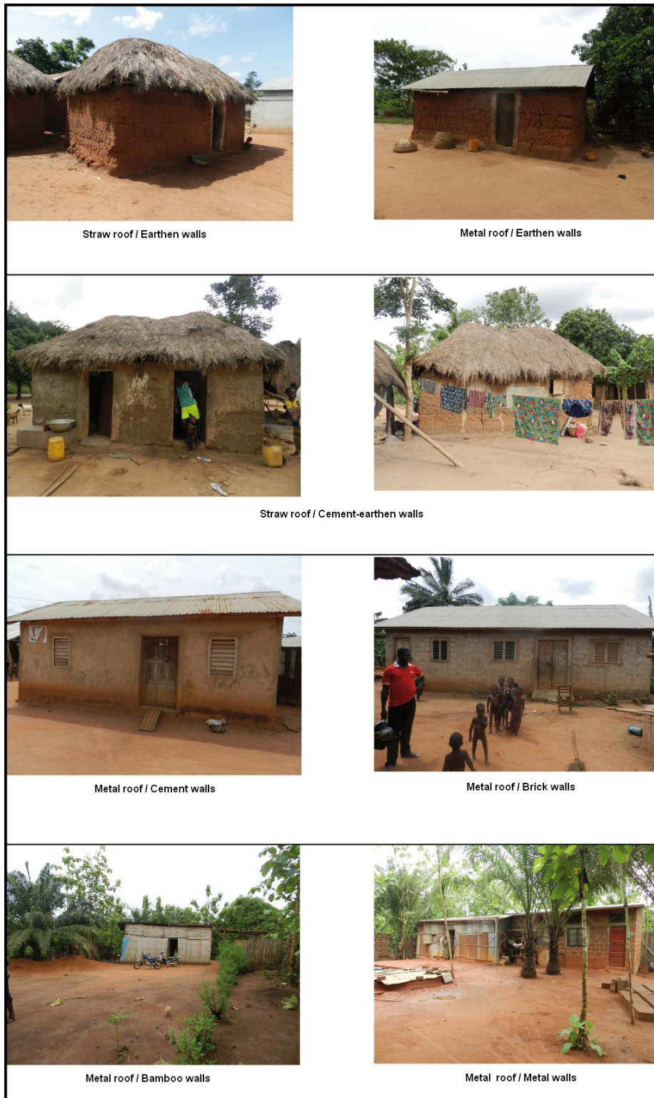
Figure 3: Diversity of the building materials used in the houses where mosquitoes were captured in the region of Allada.
